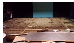
Photos from demolition of old to installation of new stage floor.
